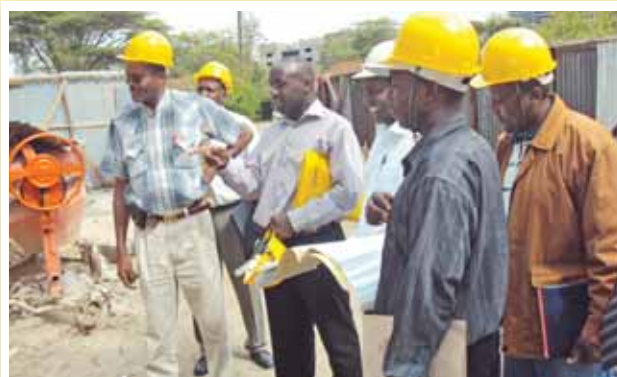
Inspection of ongoing refurbishment of the squash courts
